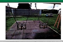
There is some wear to the shackles. - Monitor for any further deterioration and replace when 40% worn
