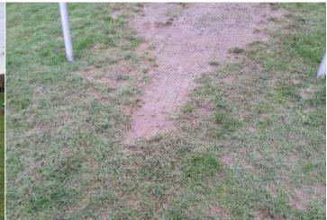
Finding: The grass mats are silted up and the soil is compacted; this may have an effect on the impact absorbing ensure the correct surface qualities are maintained for the properties of the surface
