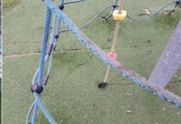
Finding: The rope has worn and wire strands are exposed Action: Replace rope or net
