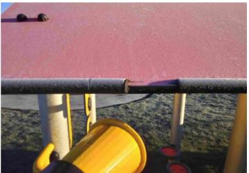
Finding: The rubber edgings are damaged or missing
